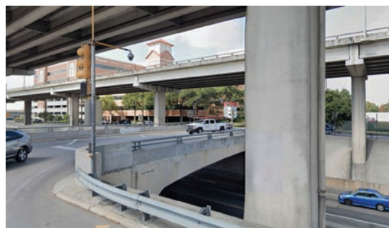
The present condition of I-35 and 32nd Street. Photo courtesy TxDOT.
